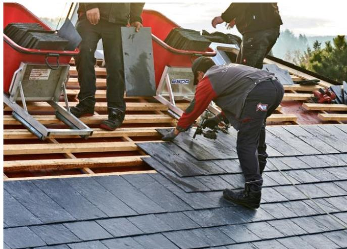
*Installation of ventilated slate roof.
